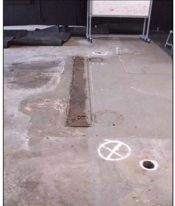
After Concrete Coring Within the Former Auto Shop (Adjacent to Former Vehicle Hydraulic Lifts)
