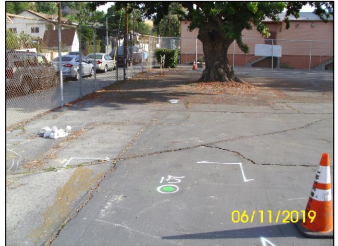
Soil Boring B15 - Location Marking Prior to Underground Utility Clearance
