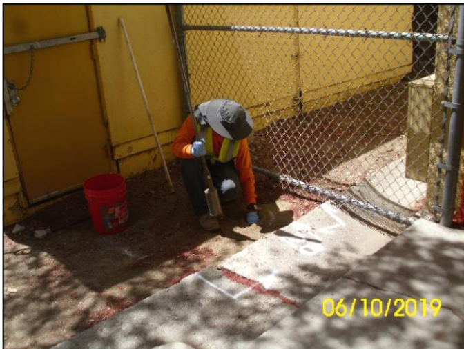
Soil Boring B28 - Hand Augering and Soil Sampling (Southwest of the Music Building)
