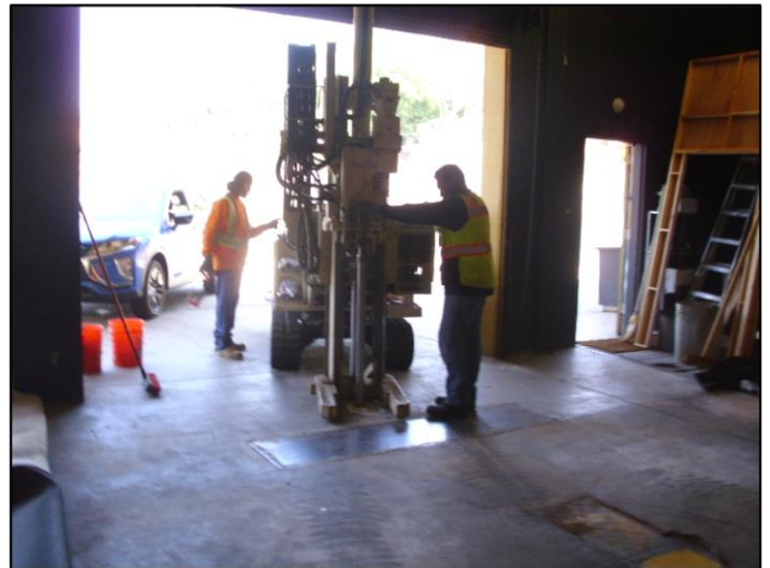
Direct-Push Drilling Within the Former Auto Shop
