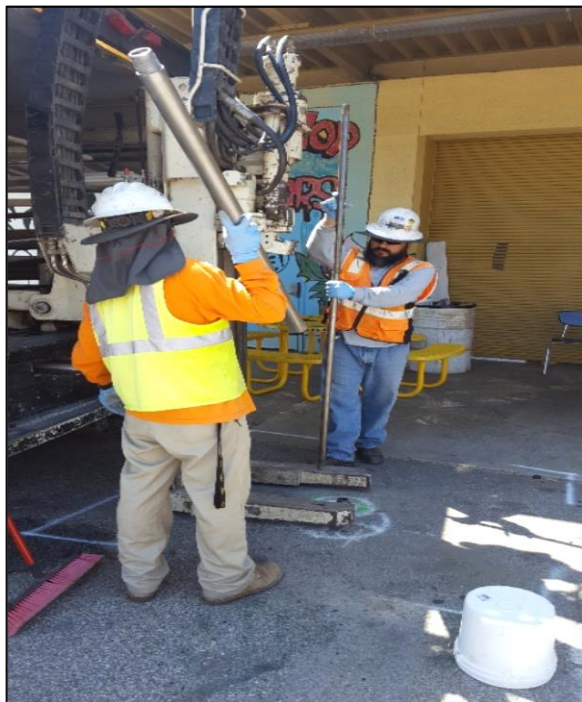
Direct-Push Drilling Within the Former Auto Shop
